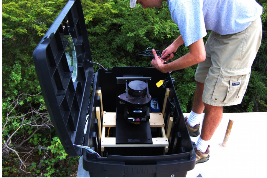
Figure B.3: Photograph of the inside of the equipment housing.
