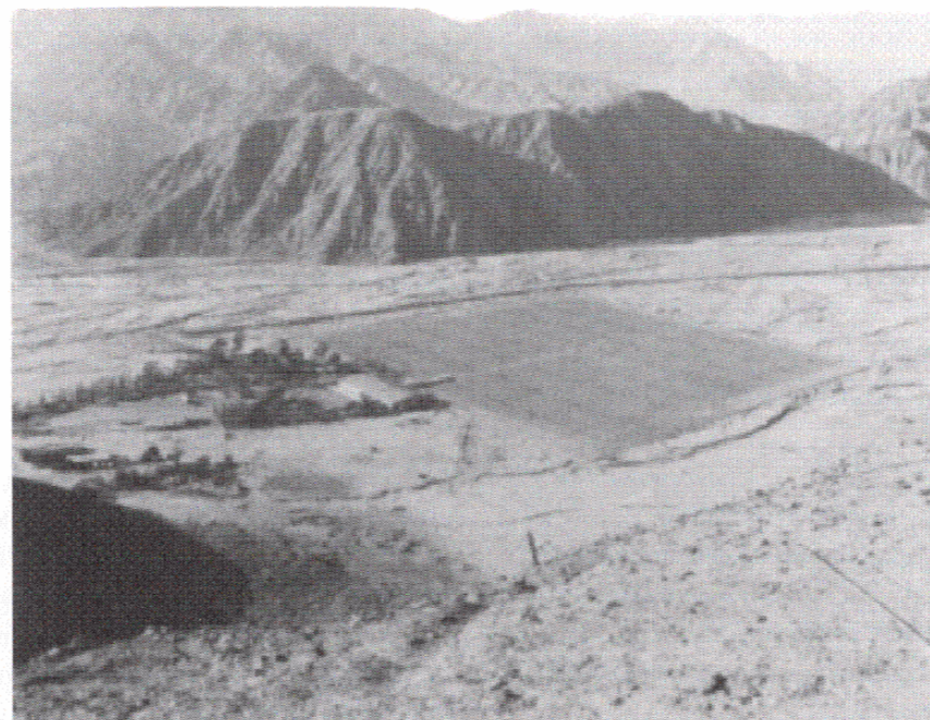
Figure 1 Panoramic view of the Jicamarca Radio Observatory and its 300 m × 300 m antenna array. The building houses a powerful transmitter with approximately 3 MW of peak power. It was the first MST radar and it is still the most powerful.
