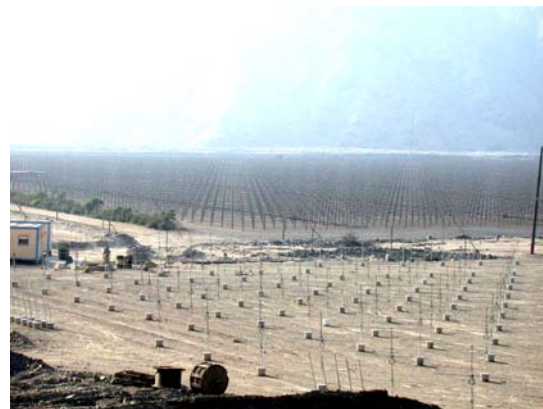
Figure 2-Partial view of the new antenna for the SOUSY radar (foreground). The large Jicamarca array is in the background.
