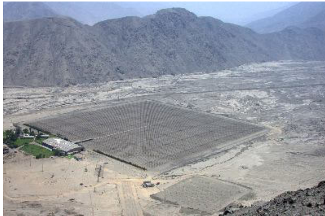
Figure 1. The Sousy Radar at Jicamarca in the foreground, with JRO main antenna in the center. The trasnmmitter and receiver trailers are in between.
